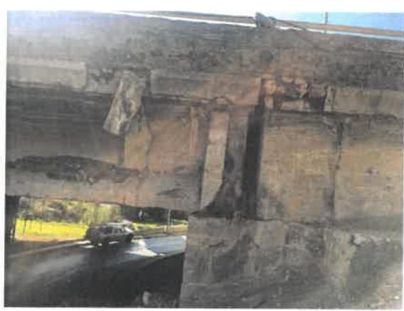
*Figure 9 Concrete Damage (Joint)*
