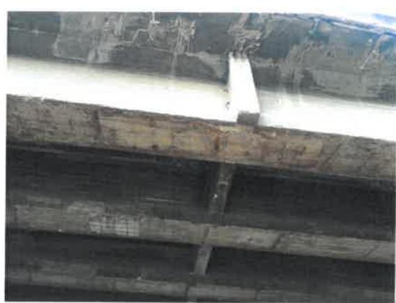
*Figure 11 Rust Appearing in the Beams*
