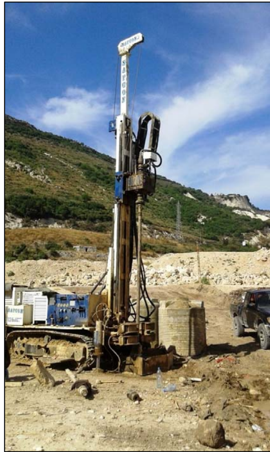
Figure 4 Crawler mounted rotary drill rig.
