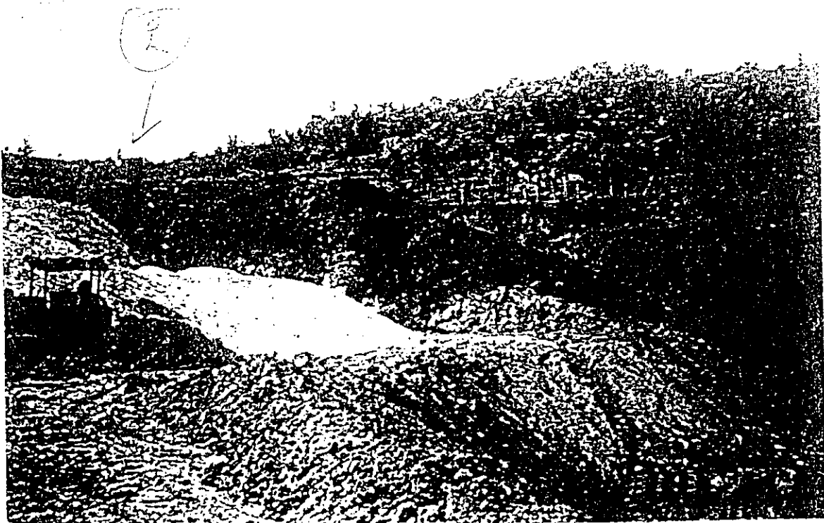
A sand source at Tannoura - Rashaya. About 60 m from houses and in close proximity to agricultural land.
