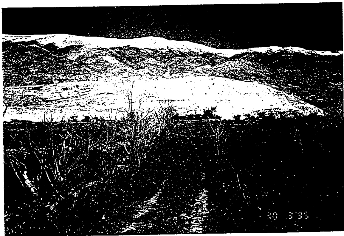
Abandoned quarry overlooking Qaraoun reservoir. It was used to build the Dam. It is benched and requires planting as it is seen from the touristic area.
